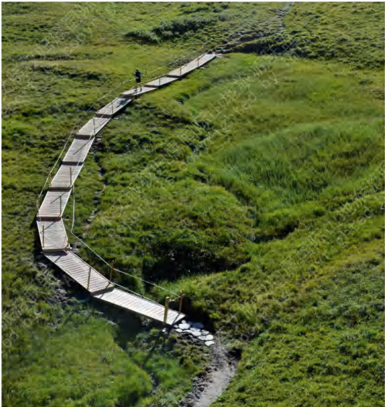
Footbridge (wooden planks) placed temporarily on the ground of a wetland for passage of hikers
