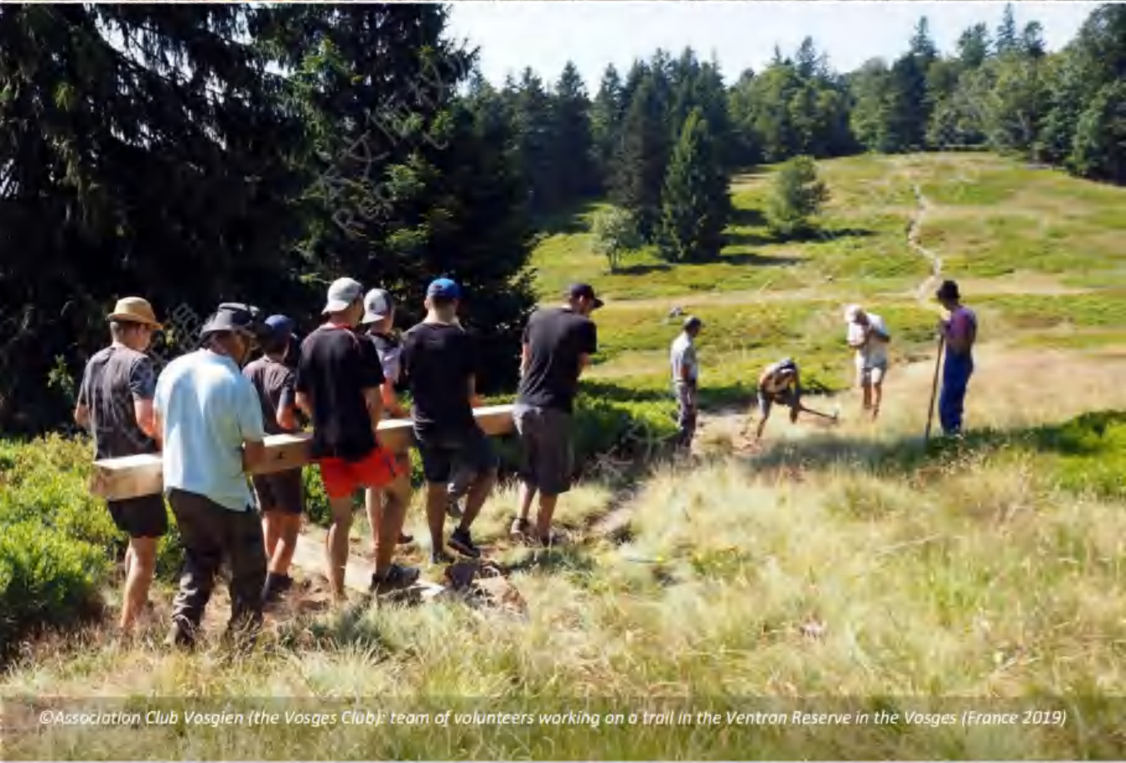
©Jules Pijourlet: volunteers working on the repair of water drainage pipes on the trails of the Tour du Mont Blanc (France)
